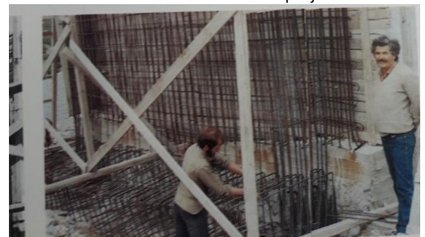
Photos taken during the works
