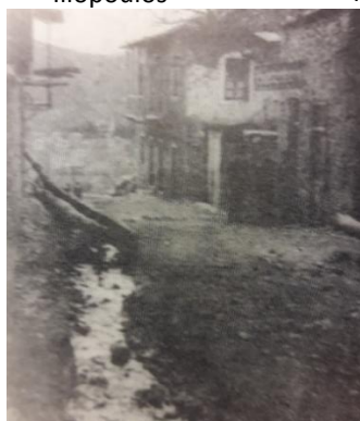
The “steno” road before the works
