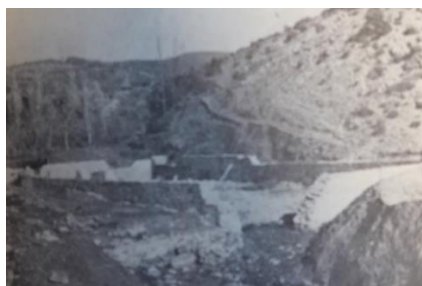
The construction of the reservoir
