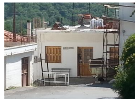
The Former Karyes' Post Office (today pharmacy)
